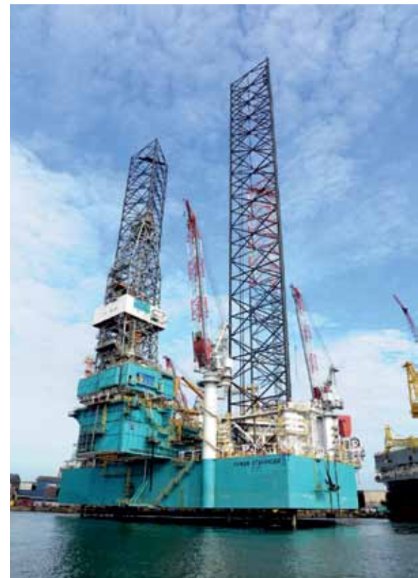
The KFELS J Class is designed as a drilling jackup rig for the Norwegian North Sea and is an enhancement of Keppel's proven harsh environment drilling rigs – the KFELS N Class (in image) and KFELS G Class
