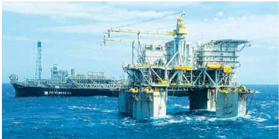
The P-61 TLWP is designed to operate with a Tender Assist Drilling Rig and equipped to receive and support work-over rig operations. It is fully outfitted and equipped for drilling, completion and work-over operations on the wells
